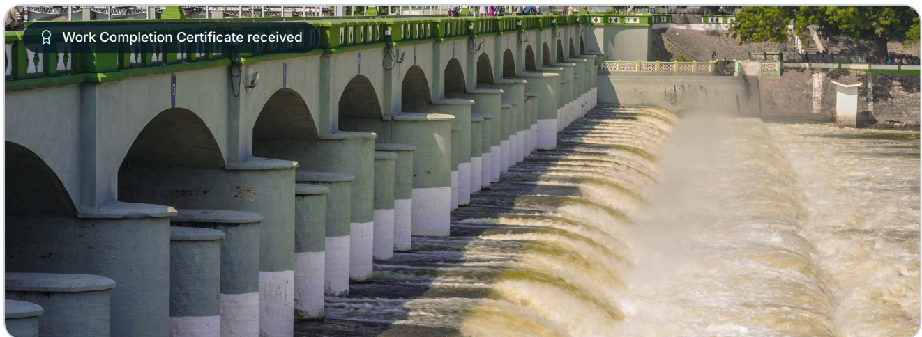
Grand Anicut (Kallanai) on the Cauvery, near Tiruchirappalli.
